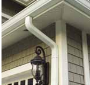
Rainware, Fascia, Soffit
